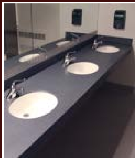
Restroom Vanity Dundalk, Maryland
